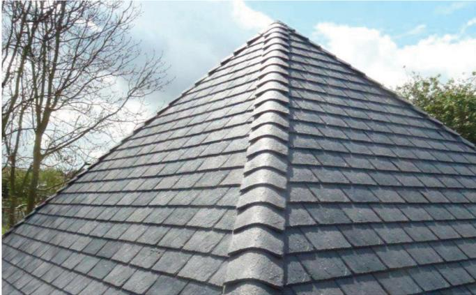
The following instructions are just a guide, and standard roofing procedures should be applied. Installers should follow guidance given in BS5534 – construction of pitched roofs (section 4), BS 5250 moisture management and ventilation and BS 8000-6 workmanship. Eco Slate is impermeable to water so requires the installation of a suitable external membrane over the sarking board.
