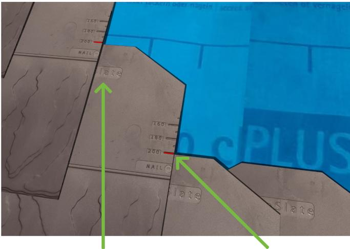
Each slate has embossed guidelines to aid location; the **vertical lines** at the top of the slate assist in locating slates horizontally.
