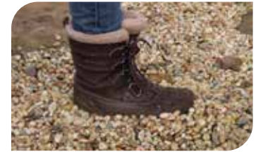
Too much aggregate
