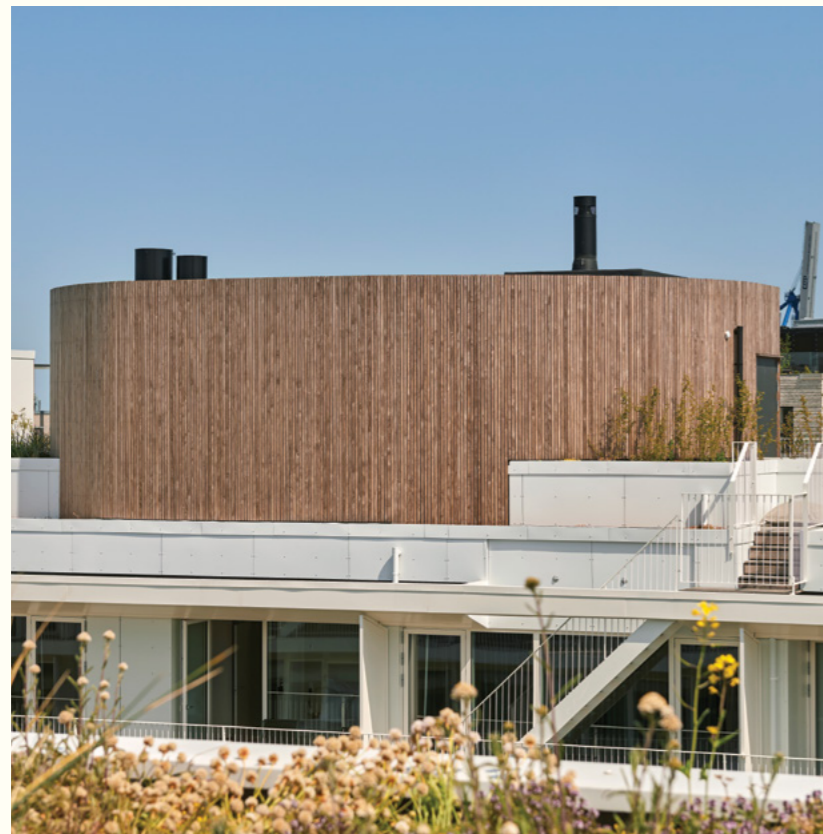
Imbue Cladding, Stubkaj, Copenhagen. Installed 2023.
