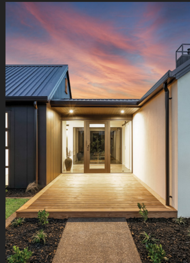
Imbue Decking, Whatawhata, New Zealand. Installed 2022.
