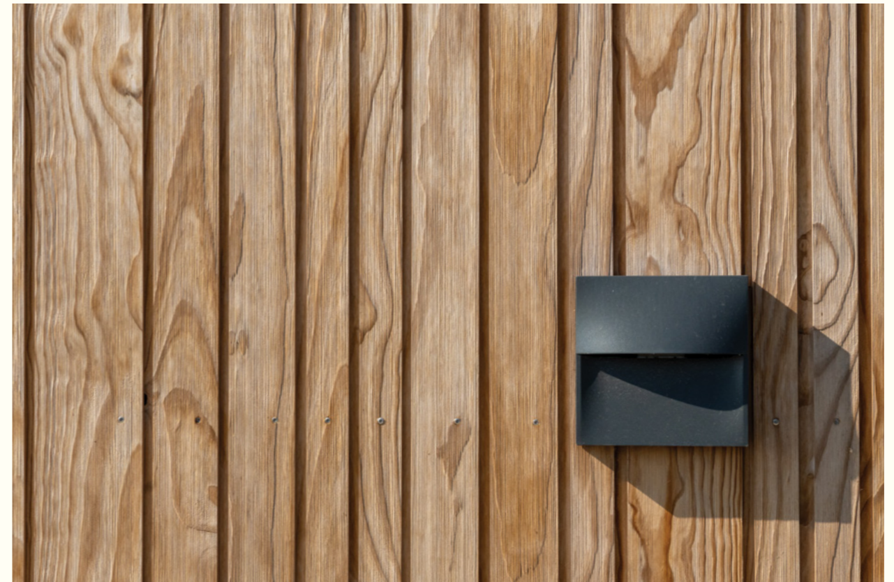
Imbue Cladding, Sydjylland, Denmark. Installed 2024.
